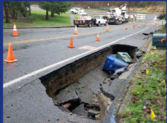
Water rates pay for the replacement of aging pipes that caused a water main break and two sink holes in January.
