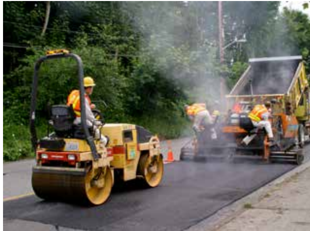
SR 7 Paving Project
