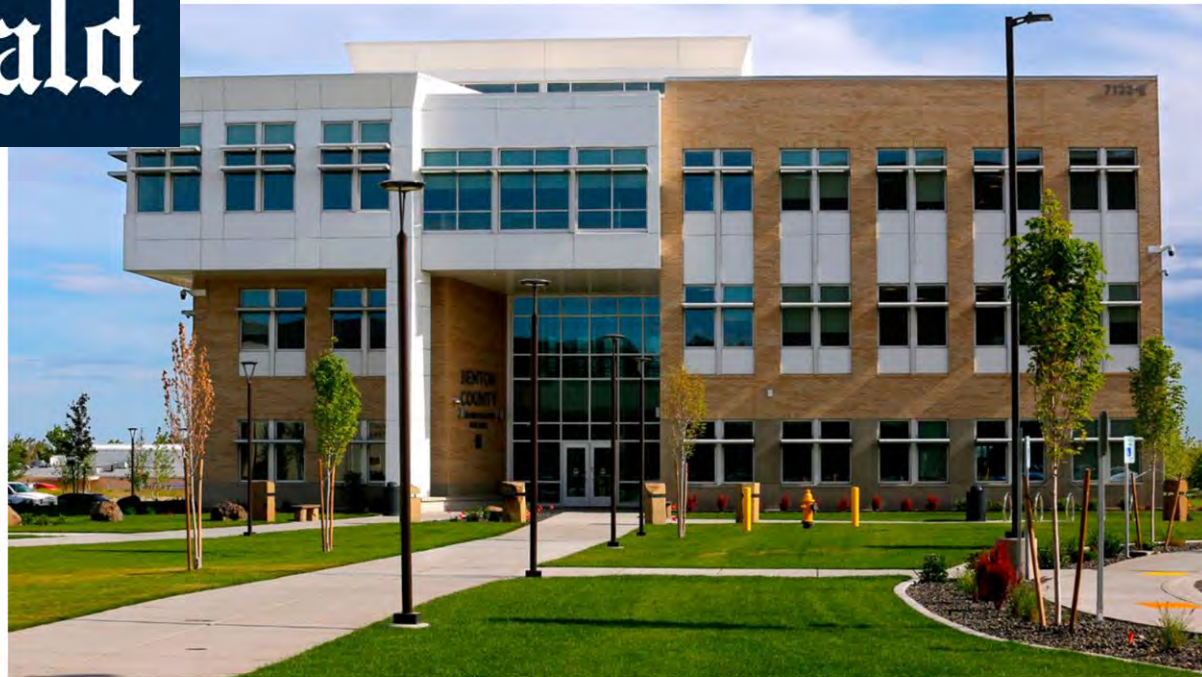
The new Benton County Administration building in Kennewick near the Justice Center. BOB BRAWDY
