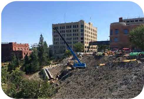
Combined Sewer Overflows (CSO)
