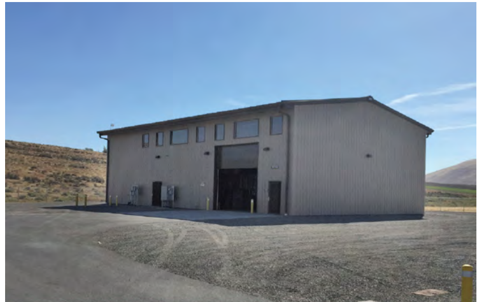
Entire plant fits neatly inside one building!
