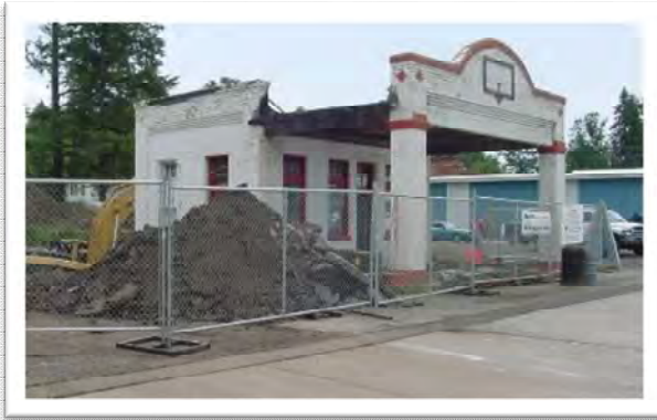
Rosalia former gas station
