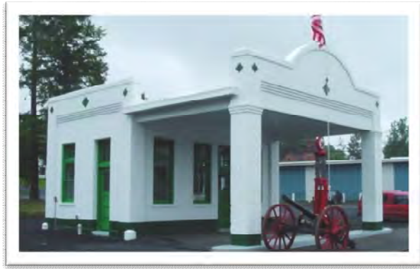
Visitors Center / Electric charging station
