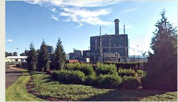
CPU River Road Generation Plant
