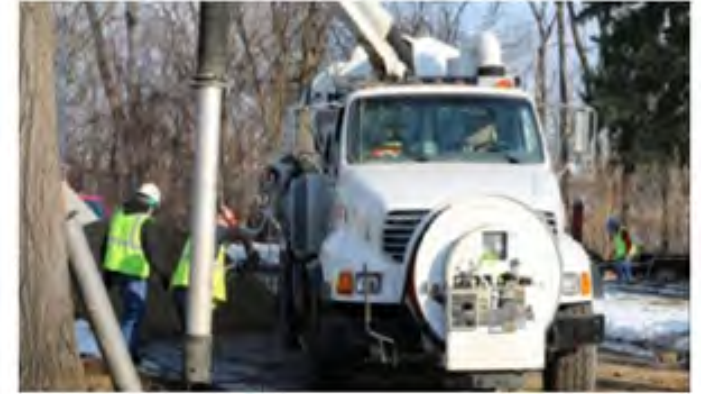
Example of Vacuum Excavation.
