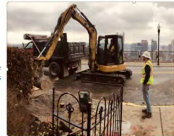
Example of a Mechanical Excavation
